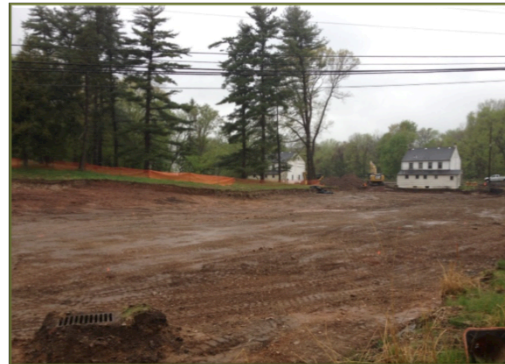
Buried asbestos waste removed.
