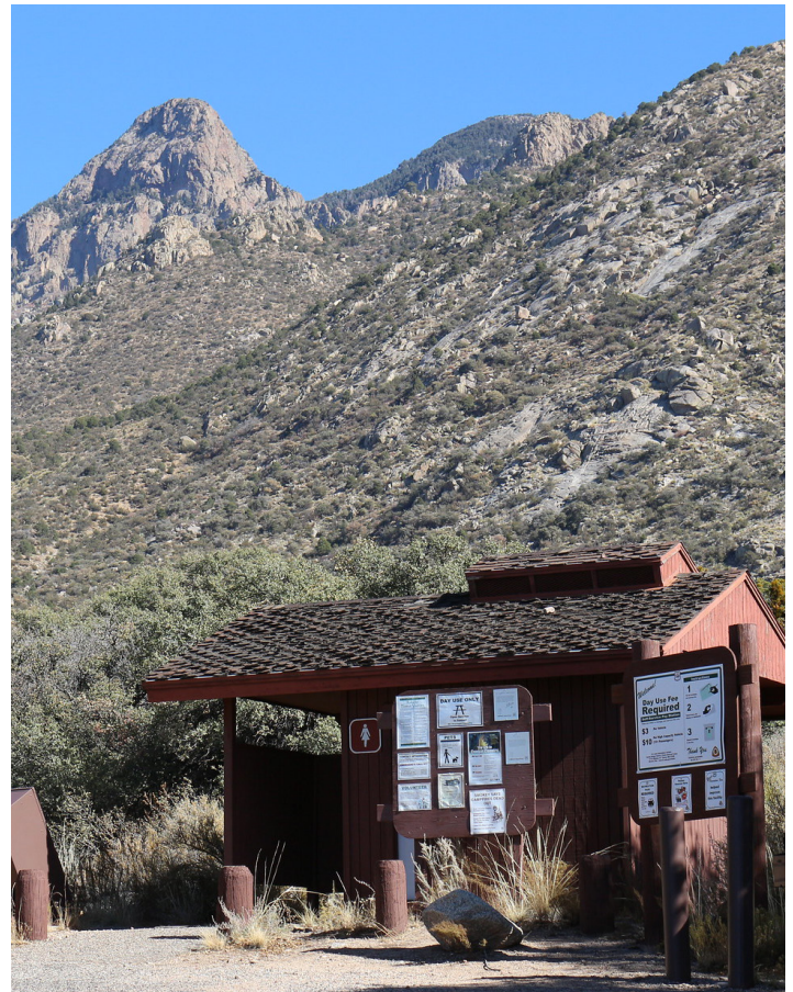
Restroom facility on the Cibola National Forest. USDA Forest Service photo.
